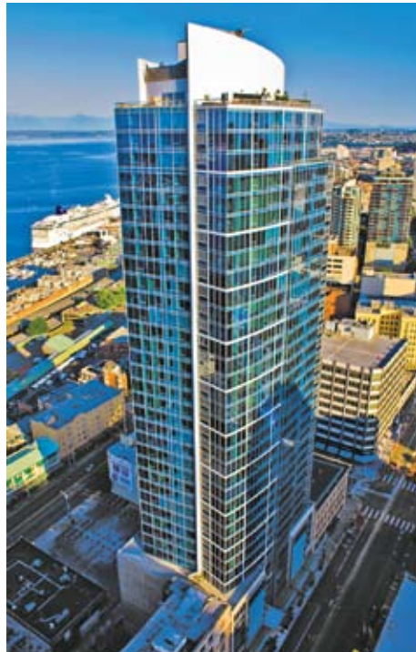
Fifteen Twenty-One Second Avenue stands 440 feet above Seattle's Pike Place Market.
